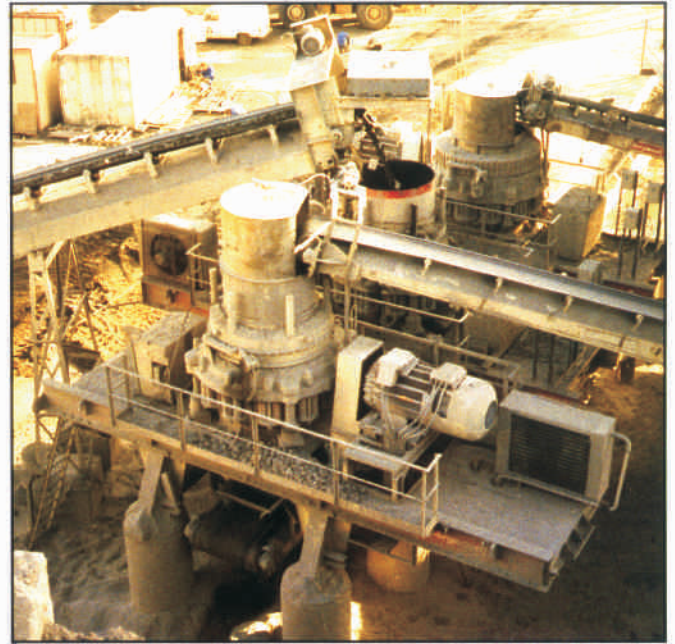
Plant with DUSTEX® in operation
